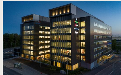
Ultimes Business Garden (Helsinki)
